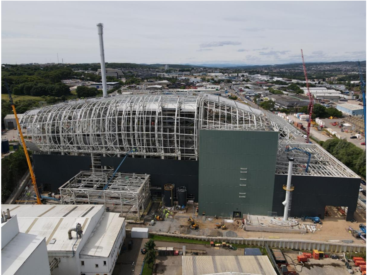
View from East of the Facility: August 2022
